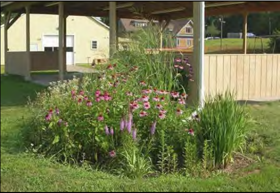
This rain garden in Vernon, CT was constructed as a demonstration project to treat and infiltrate runoff from an outdoor pavilion. Photo: USDA NRCS
