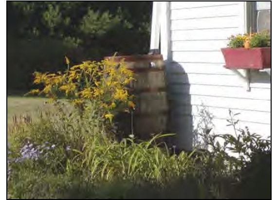
Rain barrels collect and store water from rooftop runoff for later use. Photo: P. Young
